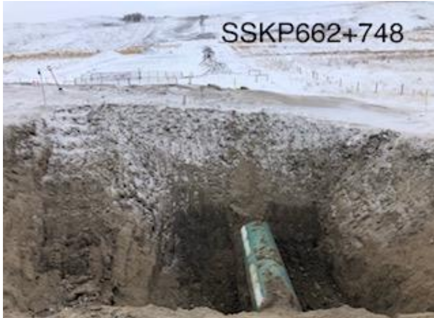
Ovality excavation east side of Vipond Creek
