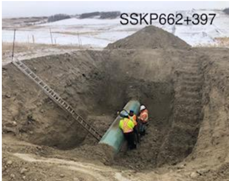
Ovality site – calliper used to check ovality
