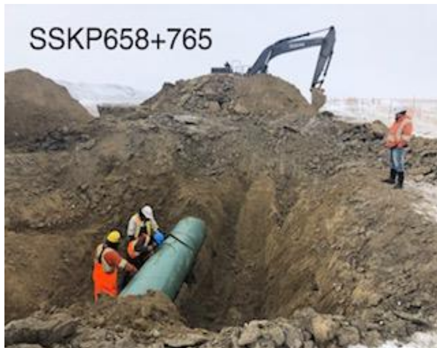
Ovality site engineer on site calliper measurement
