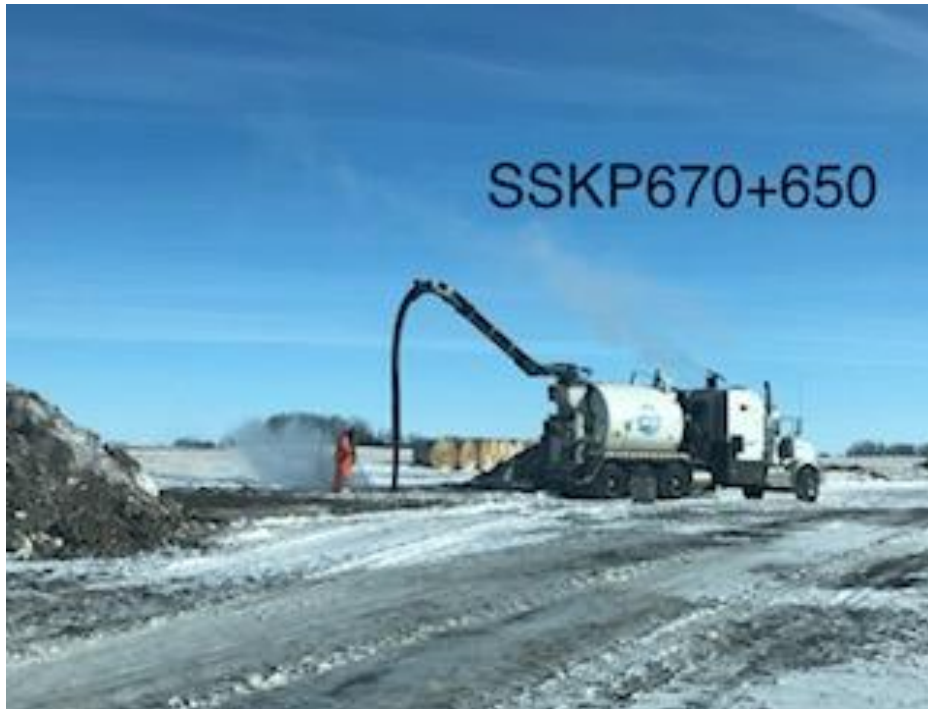
Daylighting slot trench at ovality site
