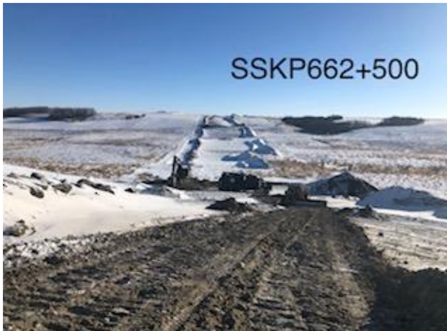
Water Course Crossing Vipond Creek SK WC72 ovality excavation
