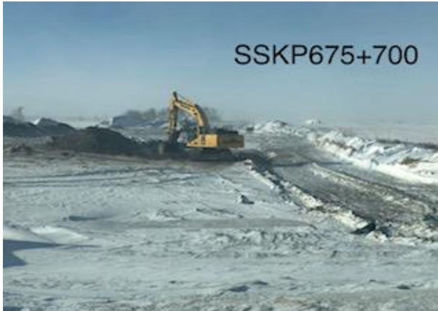
Machine clean up continues SF79 wet land crossing SK629
