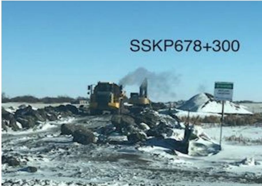
Wet land crossing ramp removal SK642
