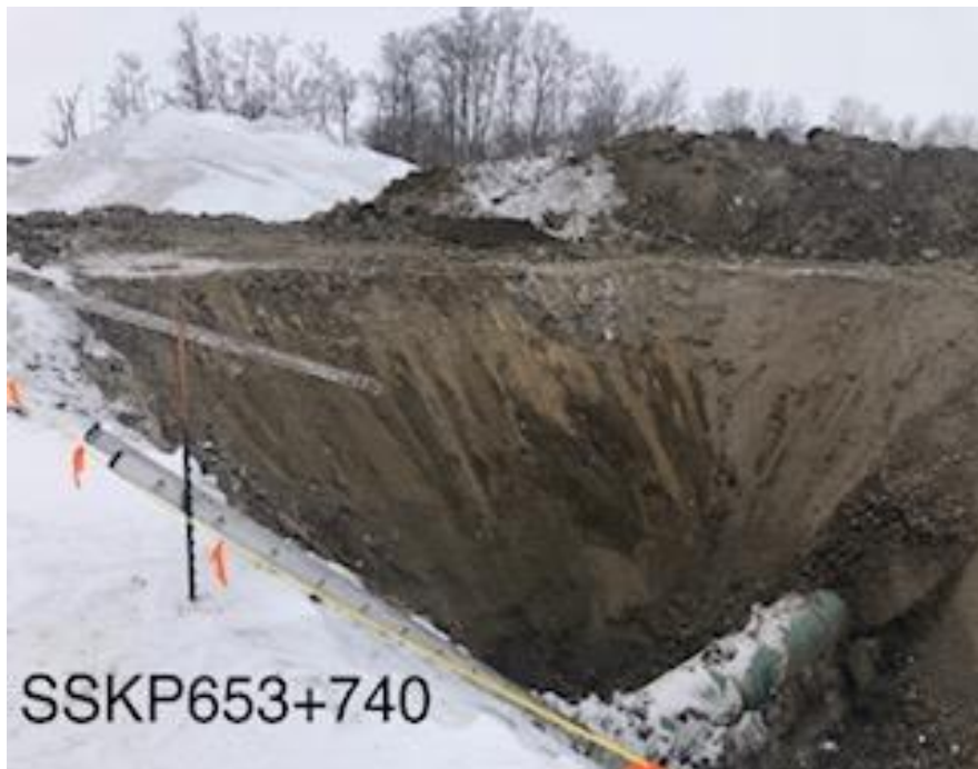
Exposed pipeline ovality site
